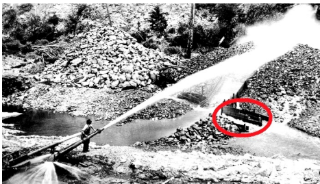
High Pressure mining: The loosened gravel would then pass over sluices (red)
